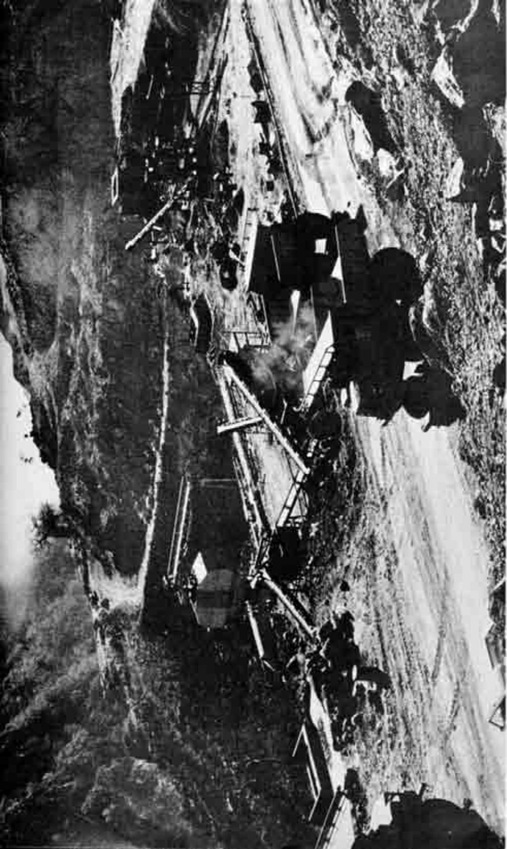
Earth movers, cranes and heavy trucks move in at Cabora Basso. Engineers are blasting a platform for the huge transformer station.
